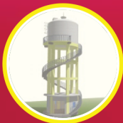
Over Head Water Tank
